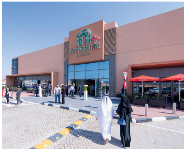
A number of sustainable measures have been implemented at the facility.
