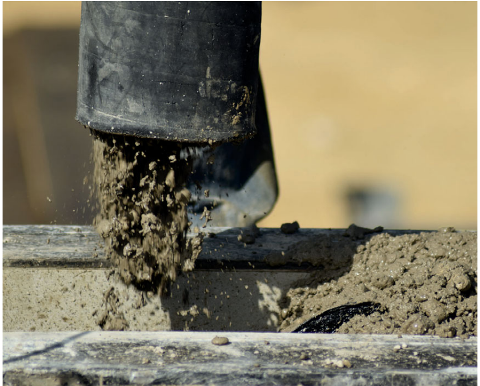
Following the completion of the acquisition, Shree Cement's aggregate capacity will increase from 29.3 MTPA to 33.3 MTPA.
